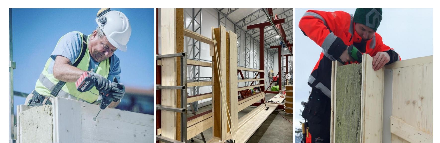
Tewo constructions are based on structural wall elements consisting of two cross-laminated plywood layers separated by insulation material and joined together with wooden dowels. The elements are prefabricated and arrive ready to be assembled on the construction site. The company is active in Norway, Denmark, the Netherlands, UK and USA.
