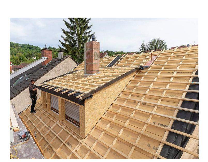
Wood-based insulation products improve the ecological footprint of buildings in two ways: the enhanced thermal insulation reduces the heating energy demand, and the nature-based raw material substitutes conventional insulation based on fossil or energyintensive products. Wood fibre insulation panels are long-lived products that can contribute decisively to transforming the building sector into a carbon sink.
